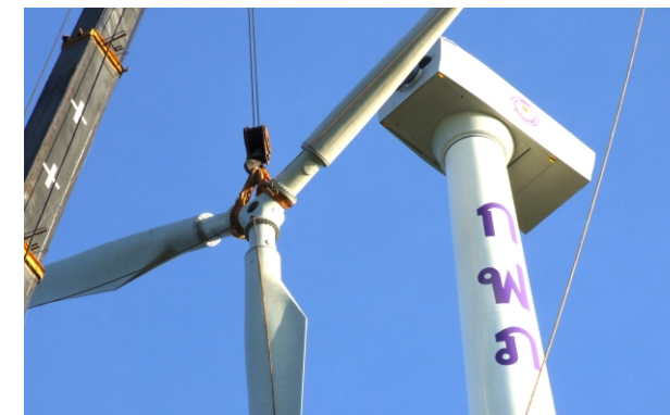
Rotor erection in Thailand
